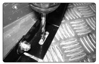
NOTE - Beware of electric cables when drilling holes
