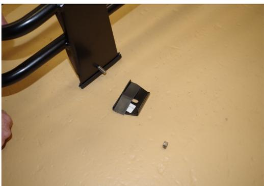
3. Insert the bolt as shown in the image above and apply the strip of protective rubber to the rear side of the bracket. This will be used to fit the legs to the guttering.
