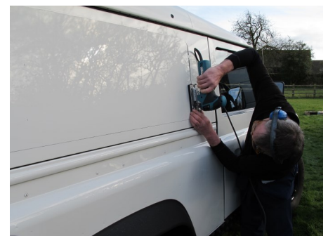
Cutting out the panels.
