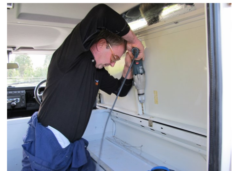
Drilling out the aperture rivet heads.
