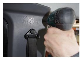
9. Secure the front edge of each side panel using two shorter screws—one in the top and one in the bottom.
