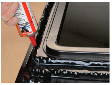
of newspaper to see that the gun is prepared and the adhesive extrudes from the nozzle right shape and thickness.
